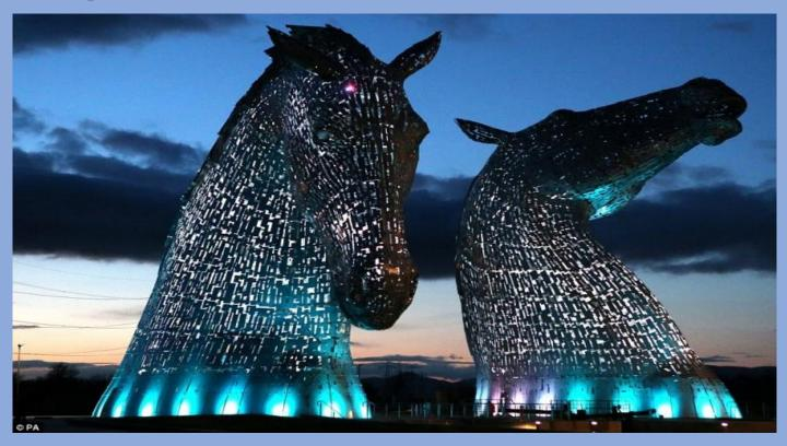
Their patterned skin, made of stainless steel, is held aloft by an intricate steel framework. At night the two statues glow in unison as the glow of upward-pointing spotlights spills out round the gaps in their surface.
